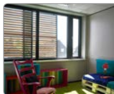
Rotating blades divided into two operating areas, which allows, for example, the blades to be open above and closed below
